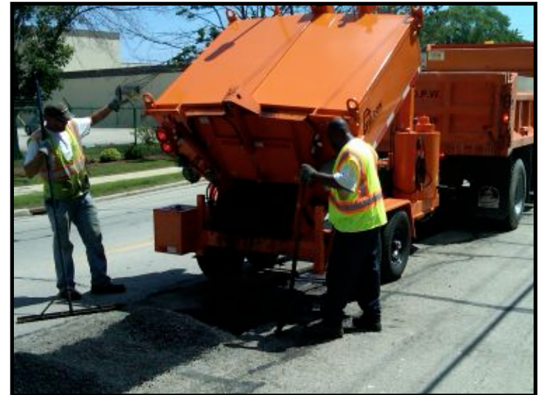
4-Ton Dump Box with Tack Tank, Solvent Tank and Hydraulic Doors Offloading Recycled Asphalt
